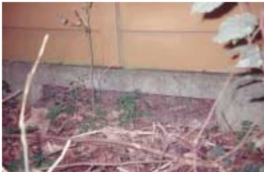
Figure 7.90 - This noise barrier has openings at the bottom to reduce the barrier effect for small animals. (Photo by H. Bekker)
