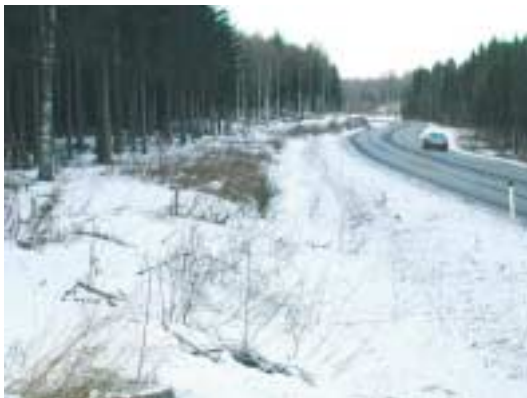
Figure 7.89 - Cutting high vegetation alongside the roads makes large mammals, e.g. moose like in this example from the E18, Akershus in Norway more visible to drivers, and removal of vegetation which is an attractive food-source will reduce the risk of having animals foraging along the road. (Photo by B. Iuell)
